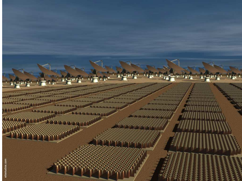
Figure 1.: An artist's conception of a SKA station. The Aperture-Plane Phased-Array occupies a large area, with many small receiving elements viewing the sky directly. This technology provides a very large field of view, and digital technology permits a large number of synthesised beams to fully sample the field of view with high spatial resolution. (image by Xilostudios)
